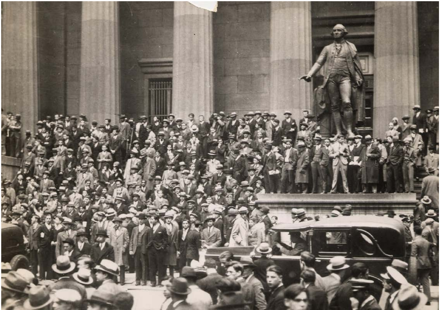
Throng at the steps of the subtreasury building (now Federal Hall) across the street from the New York Stock Exchange, October 1929.
